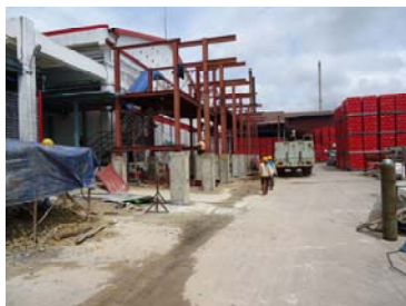
Pipe Bridge Foundation
