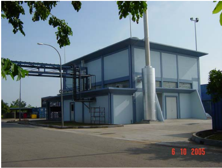
CBL-Generator Building (2MW), Container Yard, Empty store and Roads Project Robos Angkagne, Kien Svay, Kandal Province Owner: Cambodia Brewery Limited
