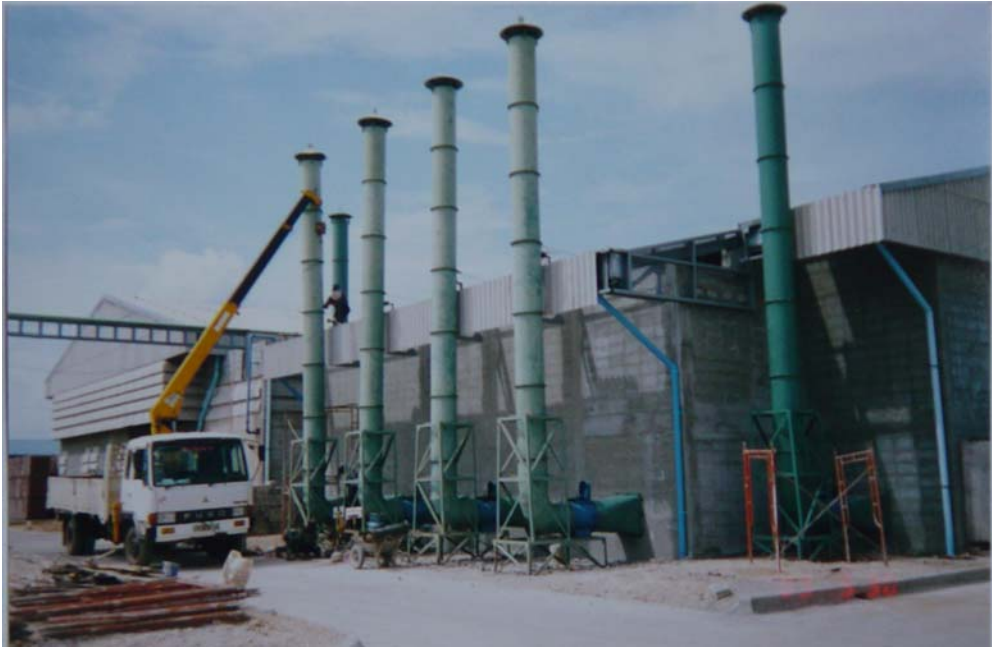
CPAC MONIER Curing Room Extension Odem (Ang Snuol District)
